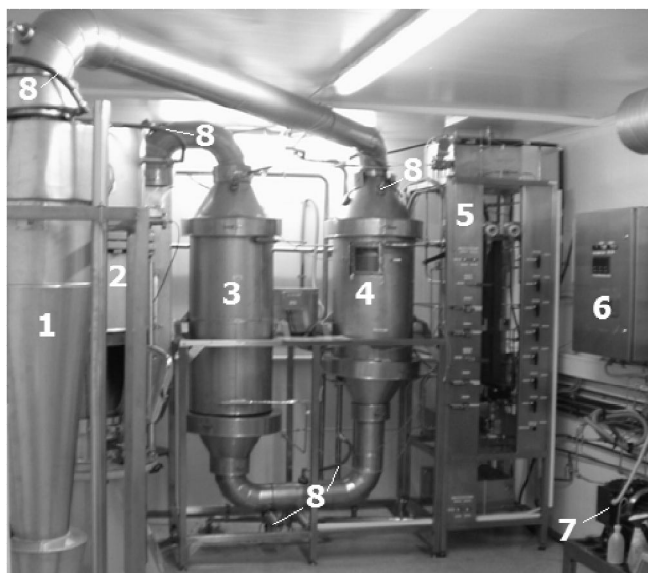
Fig. 3. The pilot scale heat pump dryer operating with R744 in transcritical cycle: 1 – cyclone, 2 – drying chamber, 3 – condenser, 4 – evaporator, 5 – adjustable external condenser, 6 – control panel, 7 – compressor, 8 – cleaning in place system.
